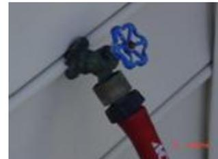
**Screw on type Hose Bibb Vacuum Breakers**
