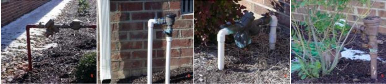
**Properly installed RP Assembly**
